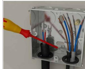
**IT MUST NOT BE CUT ALONG ITS LENGTH** as this will cause it to become unravelled. It should then be twisted back together and connected to the incoming earth on the power supply.
