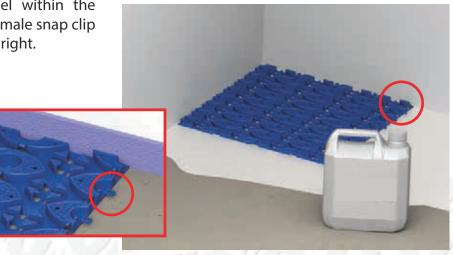
Mechanically fix the panels to the floor
