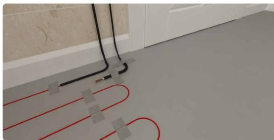
The cold tail joint can be secured in place by taping the cable either side of the joint, a small piece on the heating cable and a small piece on the cold tail. This will ensure the joint is **NOT** covered with tape.
